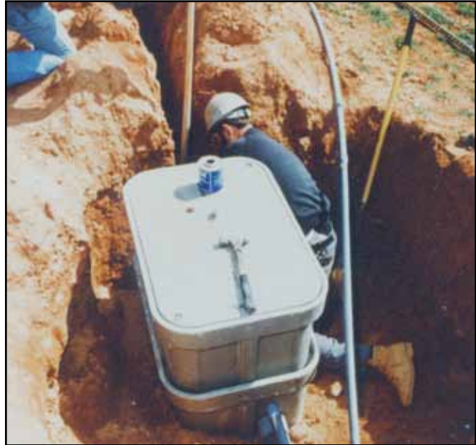
QUAZITE® enclosures are used for underground fiber optics and electric cable.
