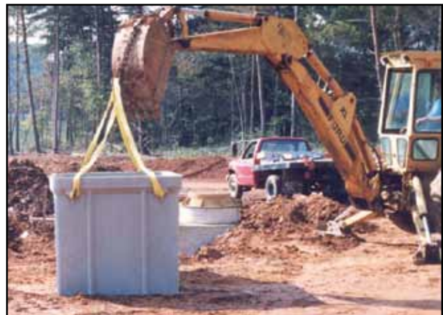
Lift and position enclosure with backhoe (4.03).
