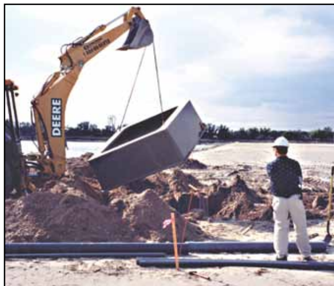
Lightweight QUAZITE® switchgear box pads (seen above) can be set in place with the backhoe used to dig the hole (precast concrete pads this size would require a crane to lift and install). The switchgear box pad also provides a large underground area with room to "train" cable into the switchgear.
